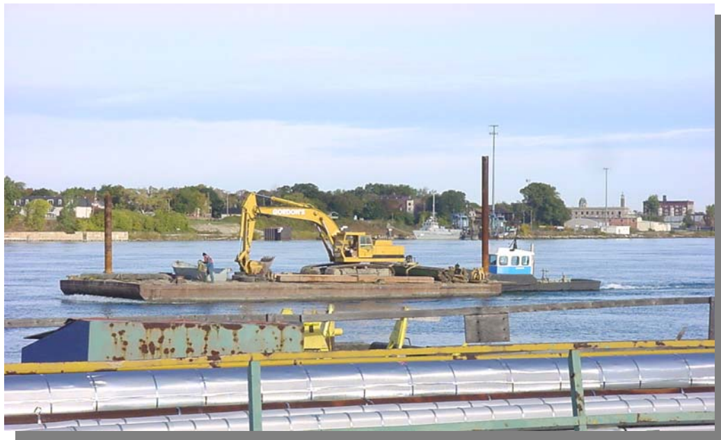
Figure 7.5: Option 3 - Excavator on a Barge, Loading Materials Onto a Second Barge to be Dumped Elsewhere
