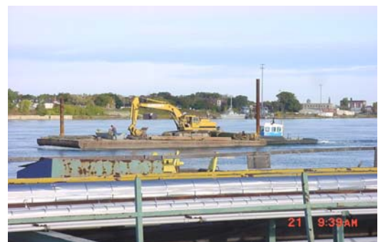
Figure 7.9: Option 10 - The combination of cutterhead suction dredging taking out loose material from the already excavated and now filled in channels, and excavation (for harder materials in main and side channels) from a barge and berm.
